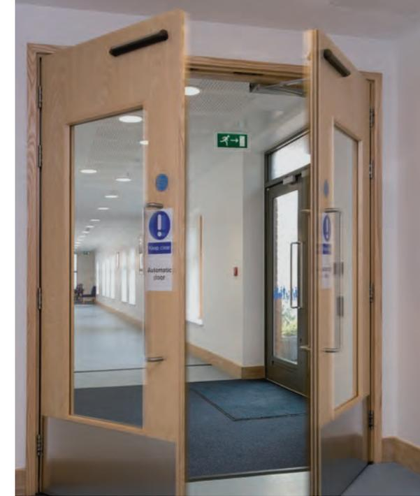
Motion sensor activated automatic operators
